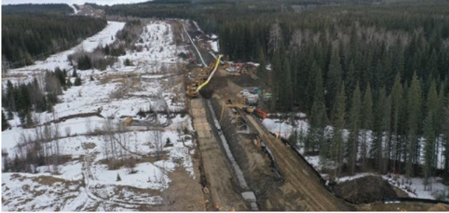
Open cut installation of the Elk River
