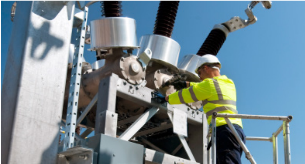
Substation work for National Grid
