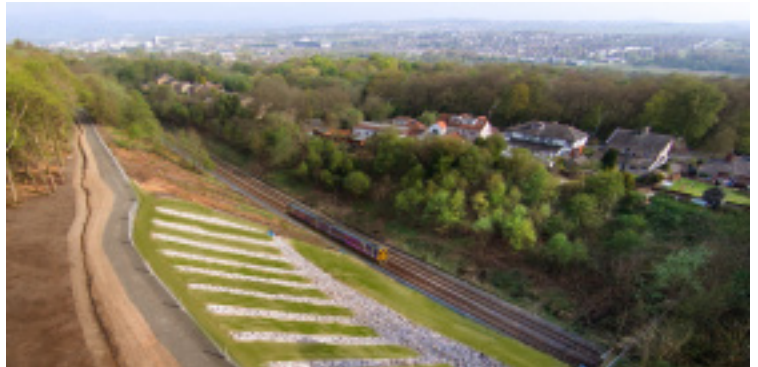
From top: Reddish viaduct, Townley tunnel, Reddish viaduct (below)
