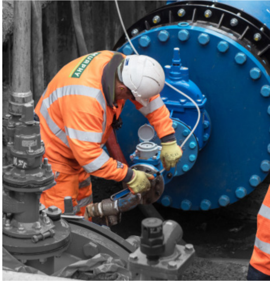
Pipeline Testing Services (PTS)
