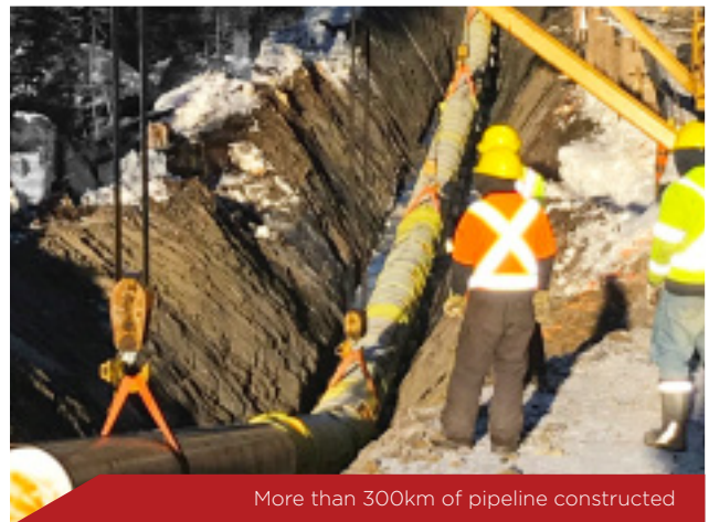
Site operatives join two sections of pipe
