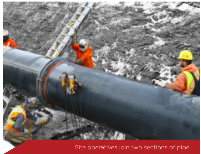
A length of pipeline is carefully laid in place
