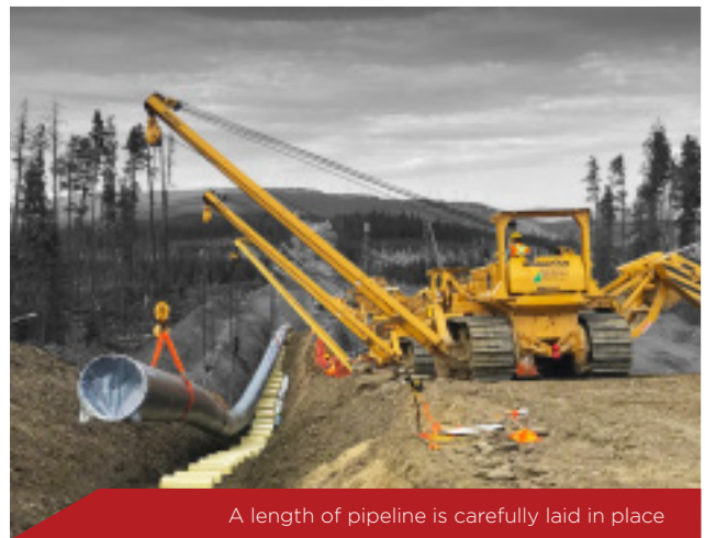
Temperatures on project fell as low as -47°C
